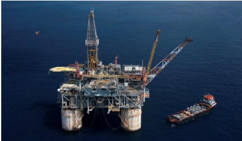
Supplying More Natural Gas
