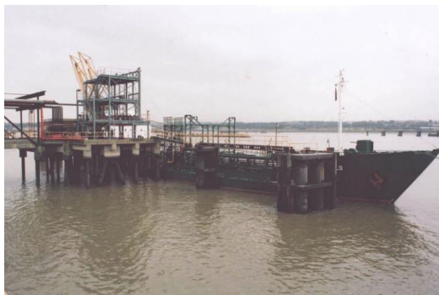
Figure 1 Barge loading operation at a petroleum terminal.
