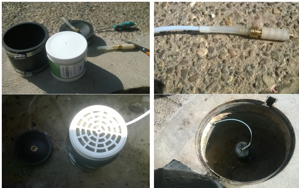
Figure 14. CO 2 trap installation.
